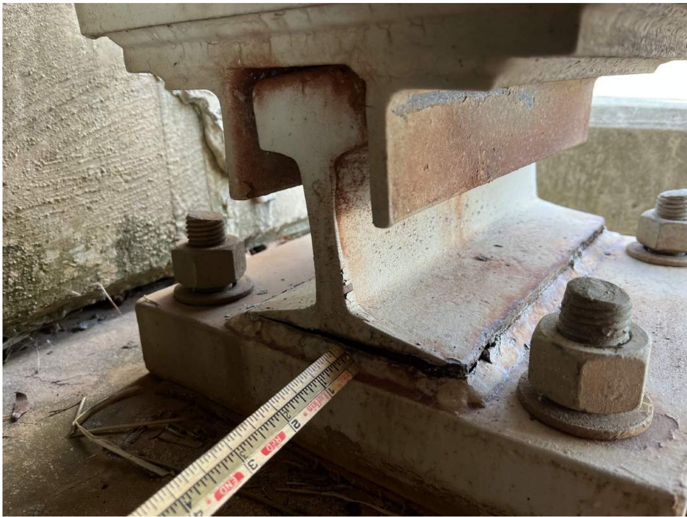
GIRDER 1 BEARING AT BENT 2
