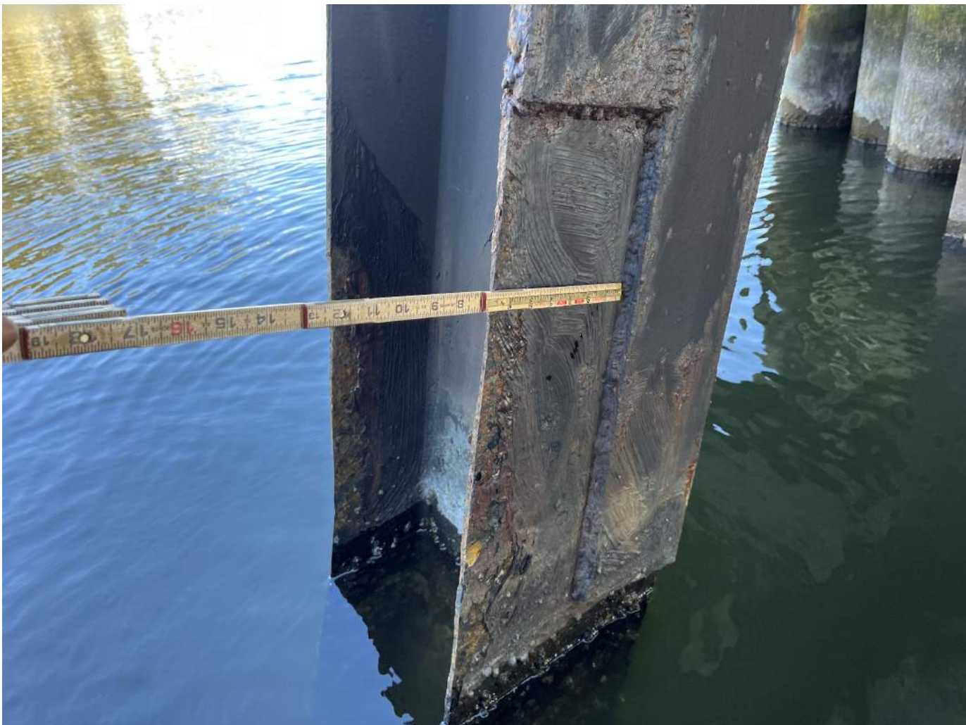
NORTH SIDE OF PILE 1
