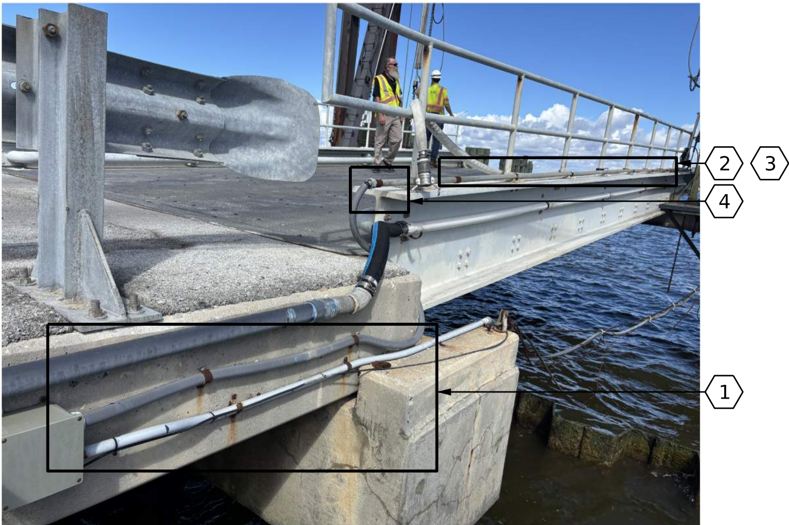
EAST PROFILE BENT 1 GATE RAILING CONDUIT SUPPORT
