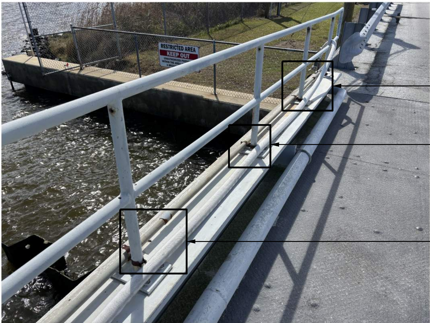
EAST PROFILE END BENT RAILING CONDUIT SUPPORT
