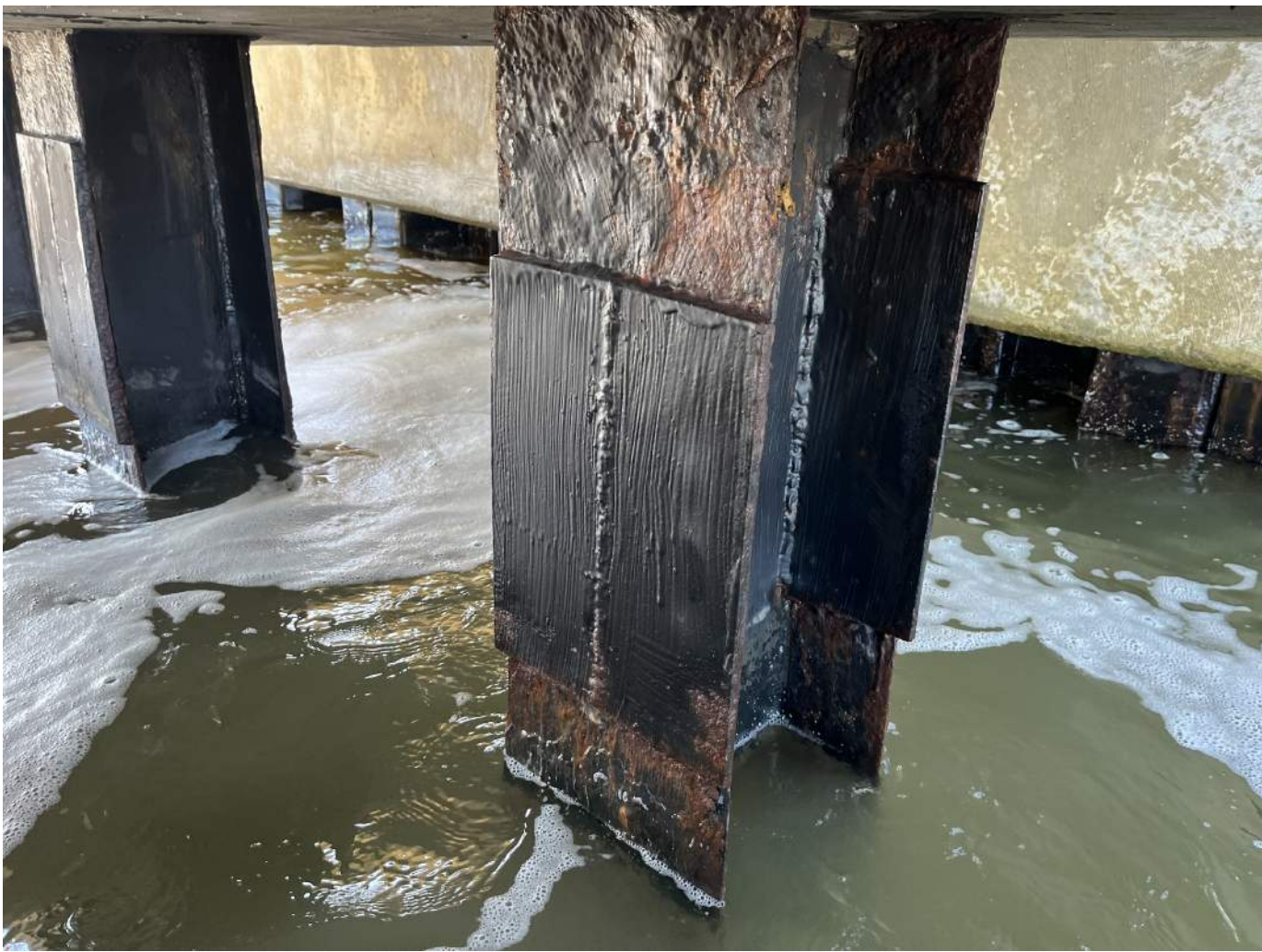
NORTH FACE OF PILE 1
