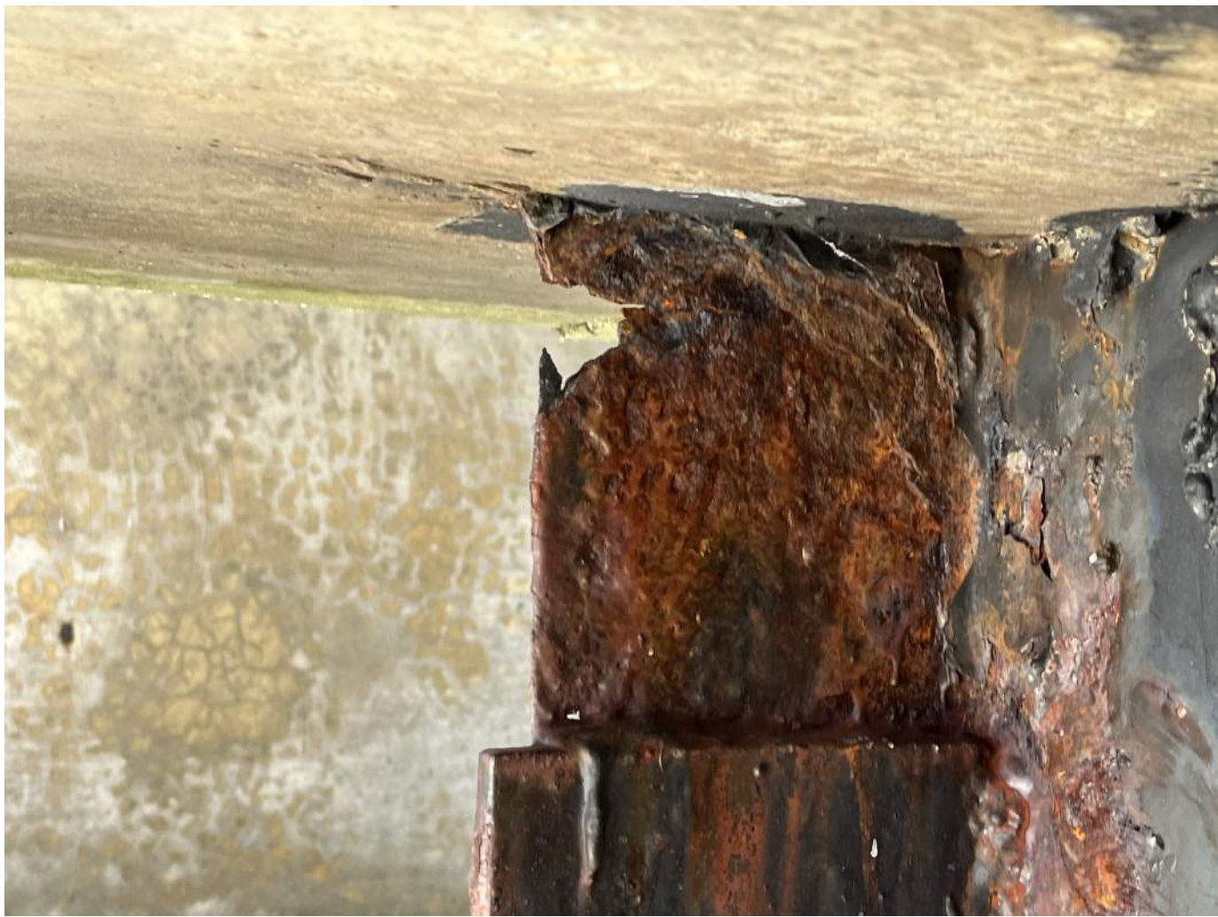
SOUTH FACE OF PILE 4
