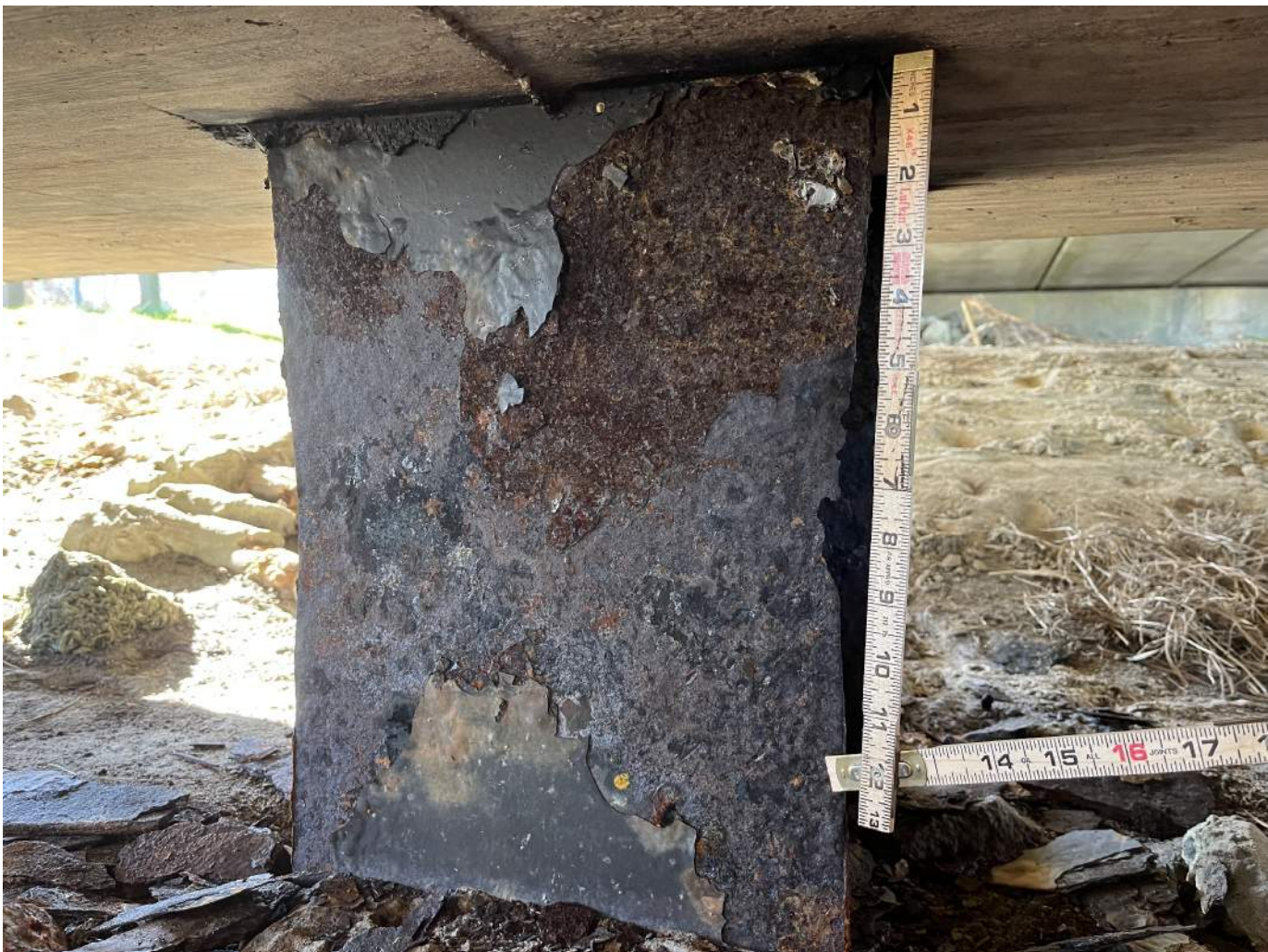
IMAGE OF PILE 3 (OTHER PILES SIMILAR)
