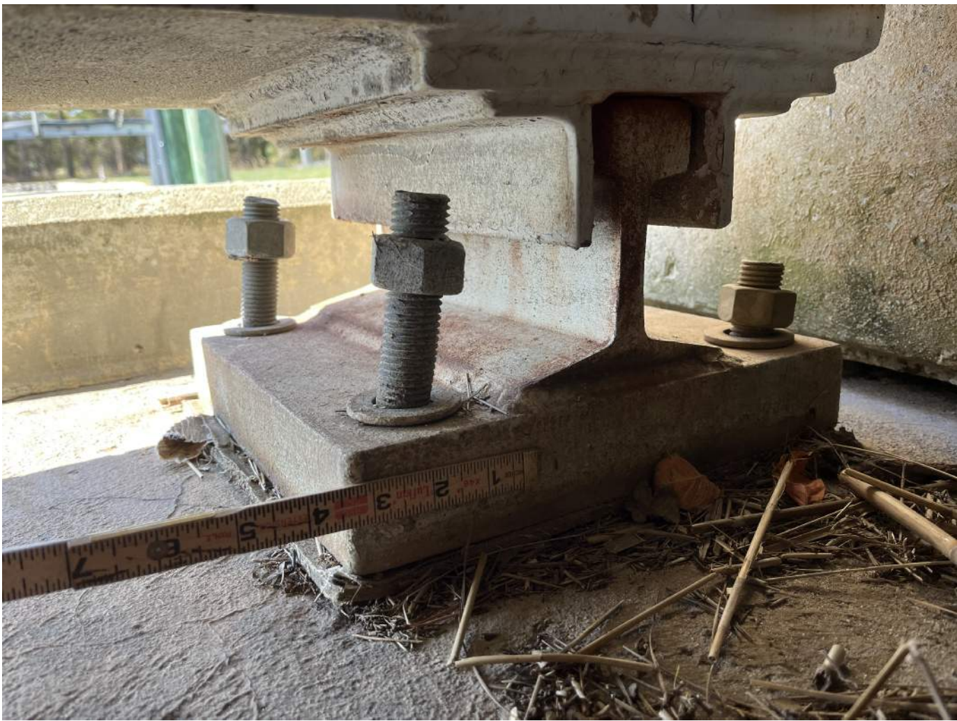
GIRDER 2 BEARING AT BENT 2
