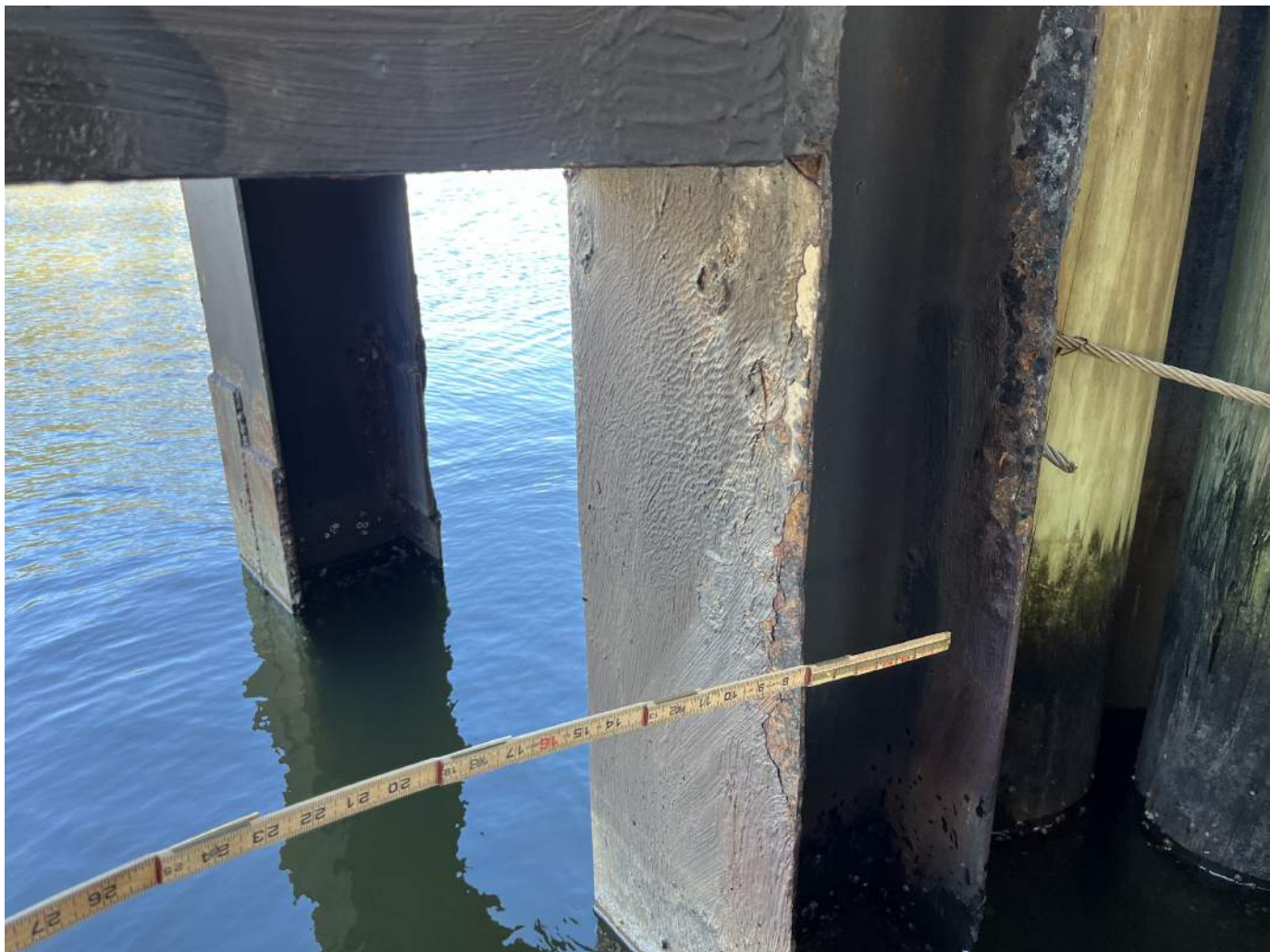
NORTH FACE OF PILE 4
