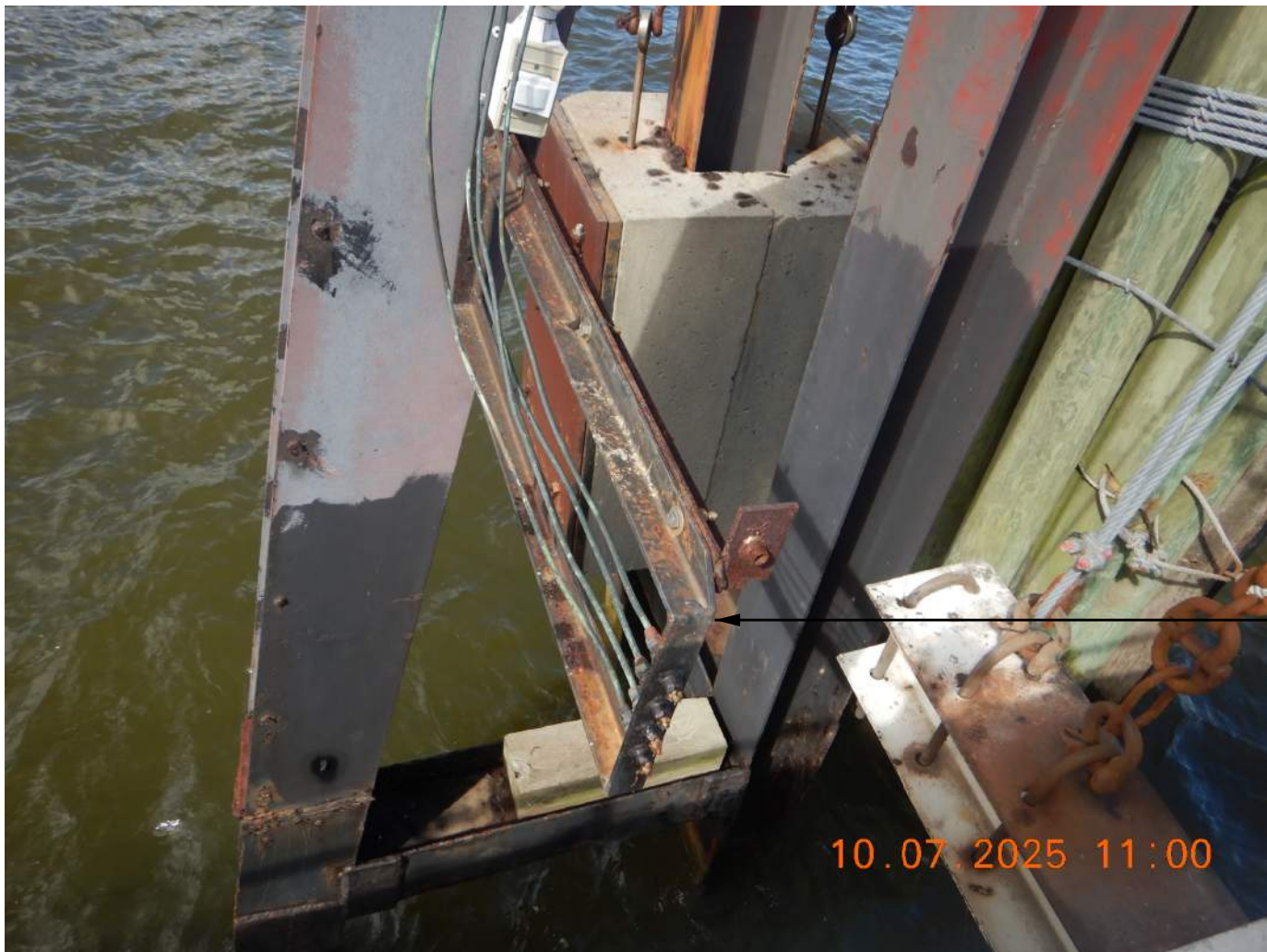
EXAMPLE LUBRICATION LINE SUPPORT MANIFOLD
