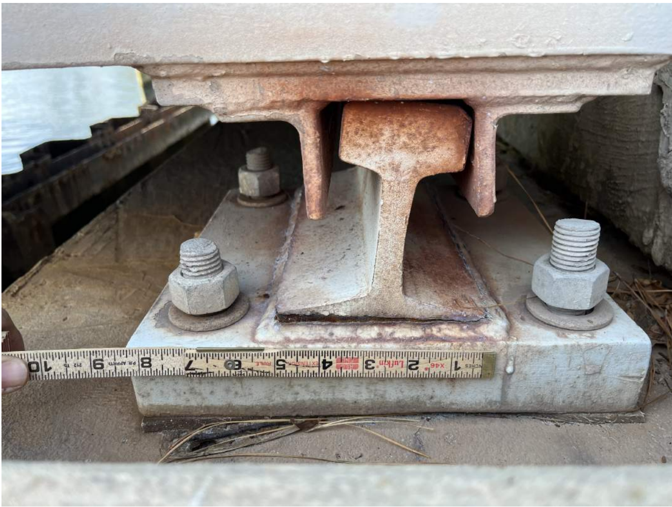
GIRDER 1 BEARING AT BENT 2
