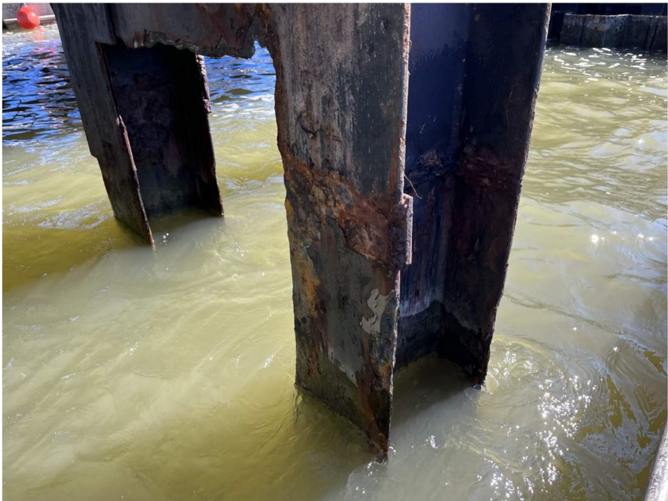
NORTH FACE OF PILE 3
