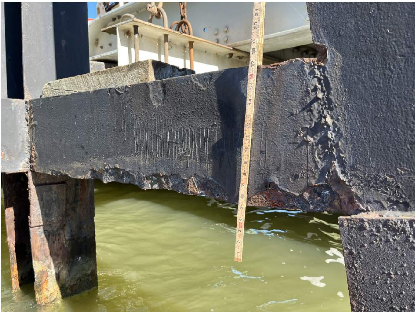
LEFT FACE OF P1-P4 BRACING
