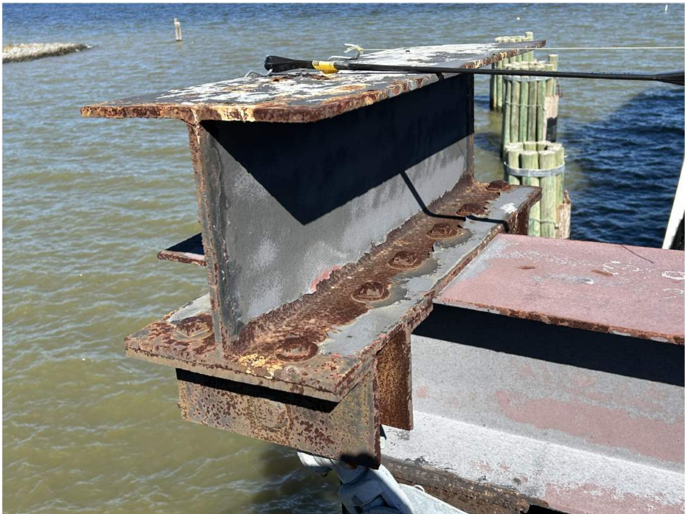
LEFT CROSS BEAM AT GANTRY CAP BEAM
