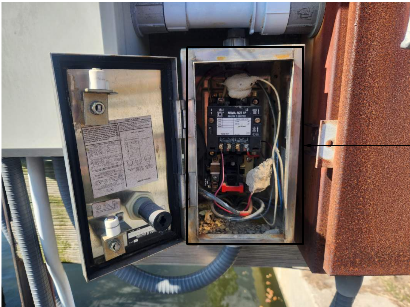
MOTOR STARTER JUNCTION BOX
