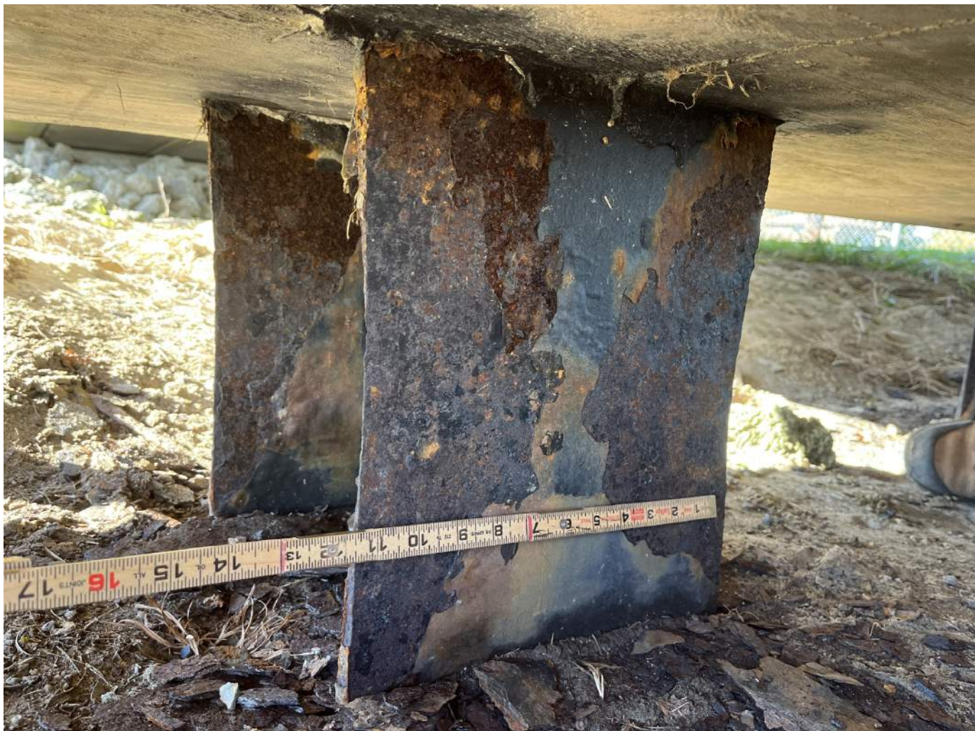
IMAGE OF PILE 4 (OTHER PILES SIMILAR)
