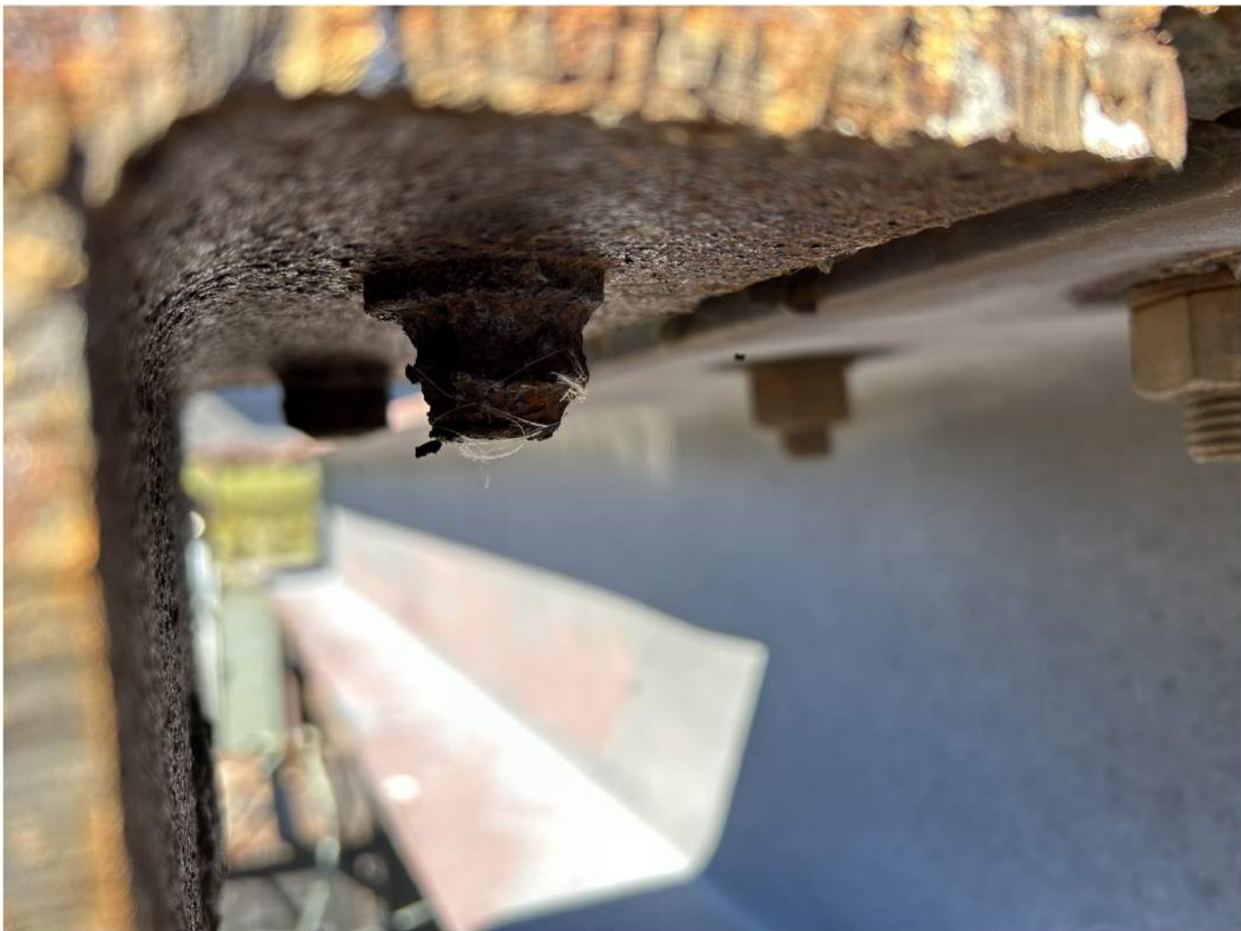
LEFT CROSS BEAM AT GANTRY CAP BEAM
